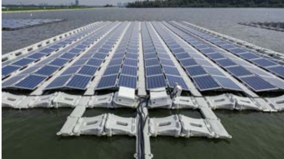
Figure 4: Floating Photovoltaic System with White Maintenance Walkway (Cision, 2017)
